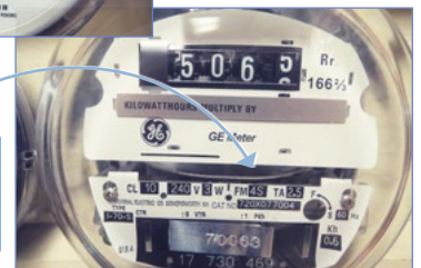
Mechanical meter: make sure this disc is spinning when system is operating.
